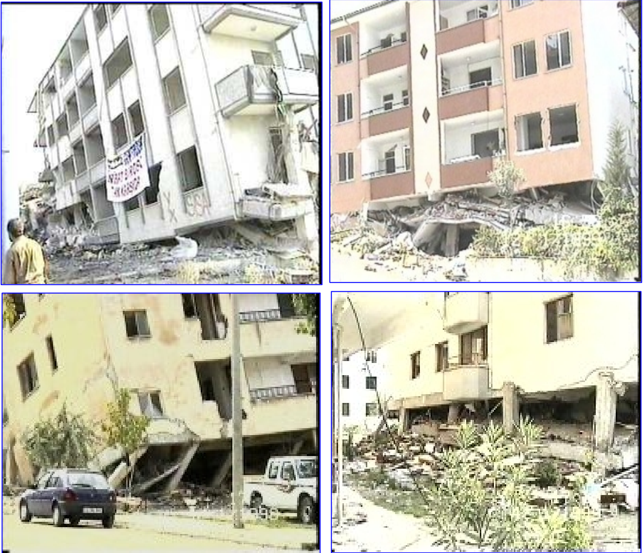
Figure 4: Damage to soft storey of Izmit Earthquake (Yalova-Gölcük)
