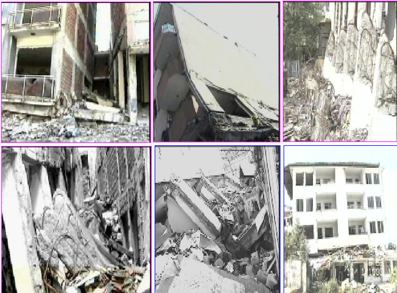
Figure 3: Damage of Izmit earthquake (Adapazarı)
