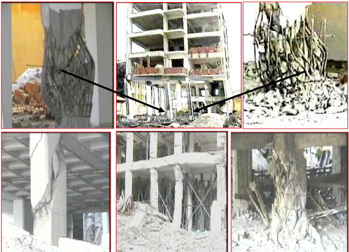
Figure 1: Damage of Izmit Earthquake (Adapazarı)
